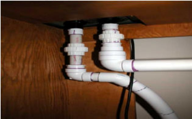
PVC UNIONS SHOWN HERE CAN EASILY BE UNSCREWED TO ALLOW SERVICING OF THE PIPING SYSTEM.
