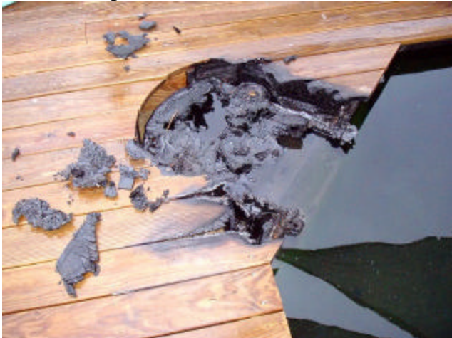
THIS SAVIO UNIT CAUGHT FIRE AND DAMAGED THE DECK TO A HOME IN WEST COLUMBIA SC
